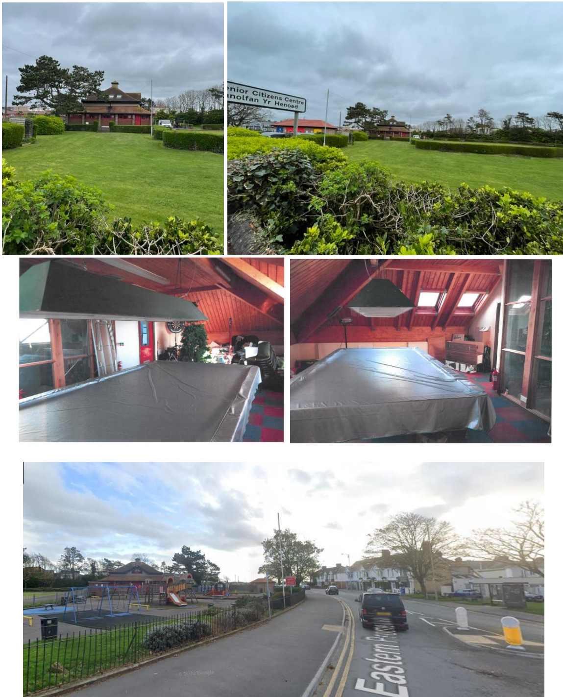
Figure 3 – Photographs and Google street view of the Application site.
